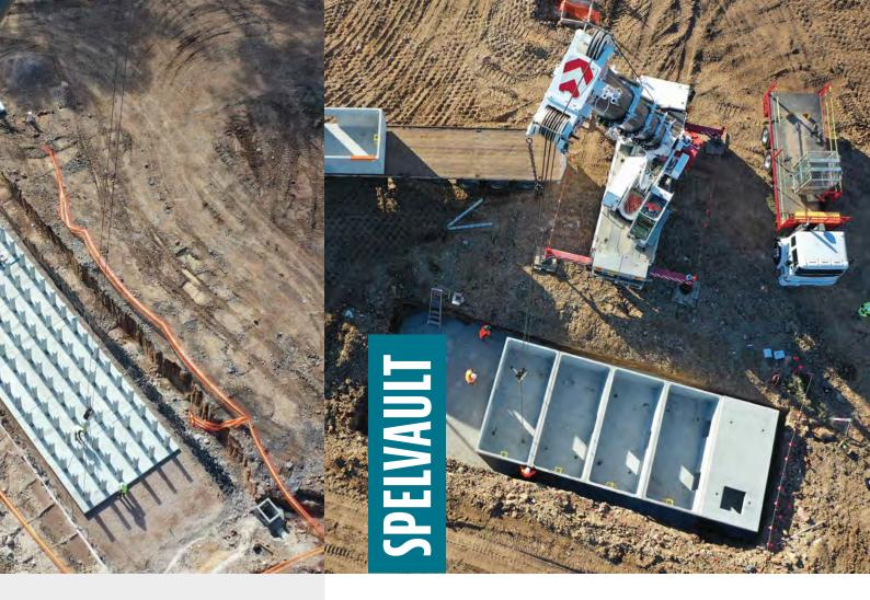
With no internal walls and precast fabrication, the design of the SPEL Megavault provides cost efficiency and easy on-site handling compared to block and slab solutions. Optimised to suit available volume and footprint, these OSD tanks are a versatile approach to flood mitigation and detention that can be tailored to fit your on-site stormwater detention requirements.
