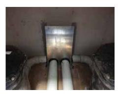
Figure 3 - Typical Outlet Weir Wall
