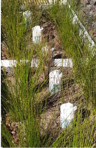
FIGURE 8. SPELBASIN® INSPECTION OPENINGS
