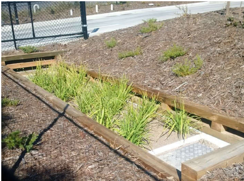
FIGURE 6. SPELBASIN® WITH TIMBER SLEEPER EDGE TREATMENT
